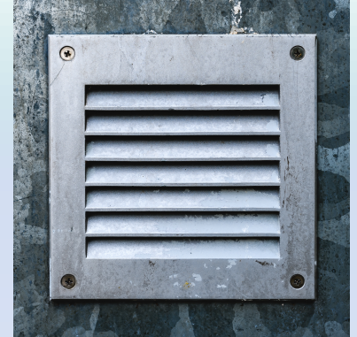
Figure 1 Typical example of a manufactured louvre ventilation system
